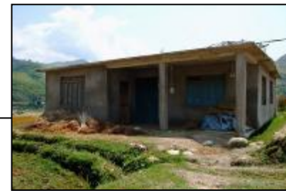
The clinic building, before our renovations.
